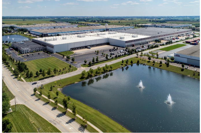
Supervalu Distribution Center, Joliet, IL
