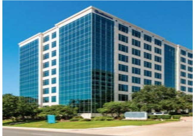
Stonebridge Plaza I & II, Austin, TX
